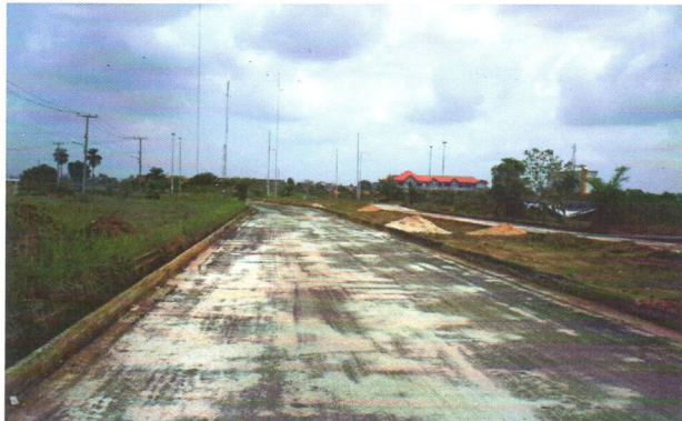
Constr. of Concord - Secretariat - PH Road (IMO)
