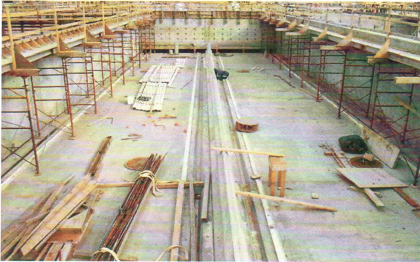
Underground Water Storage Tank
