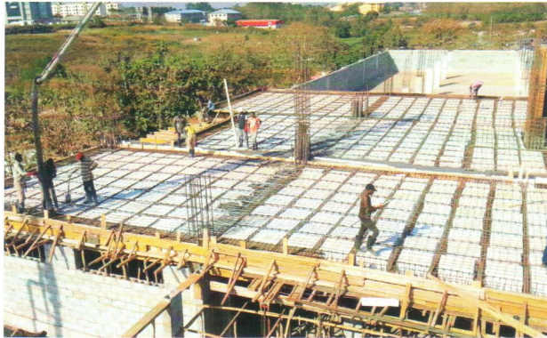
Jabi Building (ABUJA)
