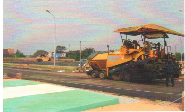
State Secretariat Parking Lots & Internal Roads (IMO)
