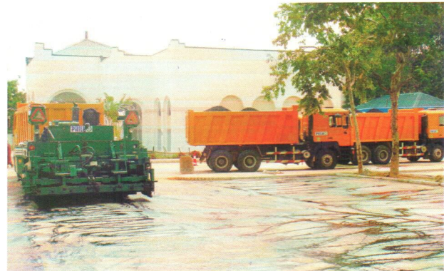
Ramat House Renovation and Parking Lot (BAUCHI)
