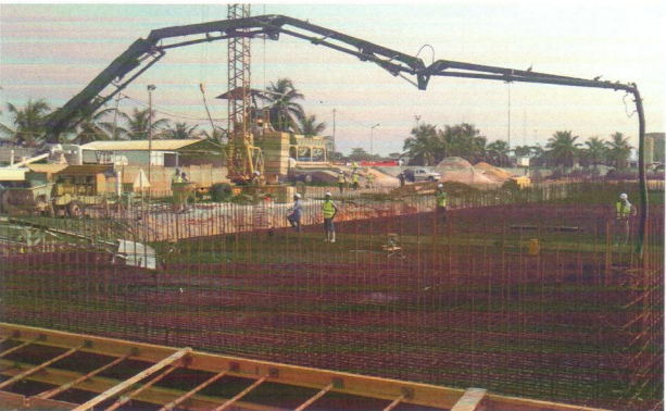
Mass Raft Foundation (LOME - TOGO)
