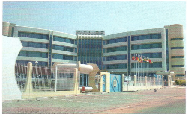
Corporate Building (LOME - TOGO)
