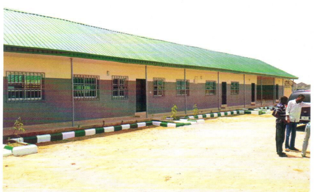
Site Offices at Ado Bayero Royal City
