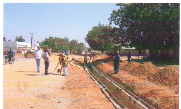
Mallam Madori Township Roads (JIGAWA)
